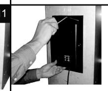
Use the self-taping screws (included) to mount the purifier to the duct .Hard-wire the purifier to the Electronic Air Cleaner Terminal or Fan Relay.
