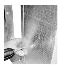
Use the included metal frame to trace the outline onto the duct (allow for a 1/4" space around the marking as to allow the frame to sit properly in the duct. This will be the guide to cut the duct opening. The duct opening is 12.25" x 6.25".
